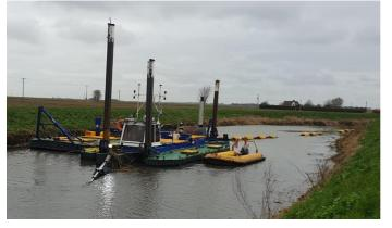
A total of 55,000 cubic metres of silt has been removed. The dredging area was extended, as more silt was found than surveys indicated. This is not unusual in a complex silt removal operation like this.
