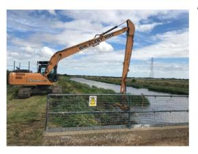
**Completing weed cutting** by mid-September using a boat and an excavator fitted with a weed rake - see photo left – to get the roots out of the middle of the river ready for dredging. Some reeds are left on the sides of the banks to help to stabilise it and prevent slips, which cause weak places. They also act as good habitat for fish.
